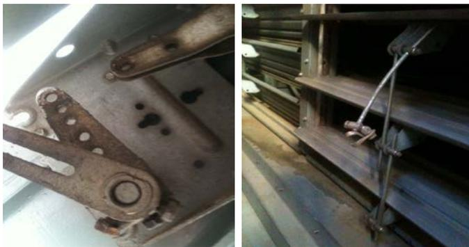
Figure 11. Common Economizer Failures
